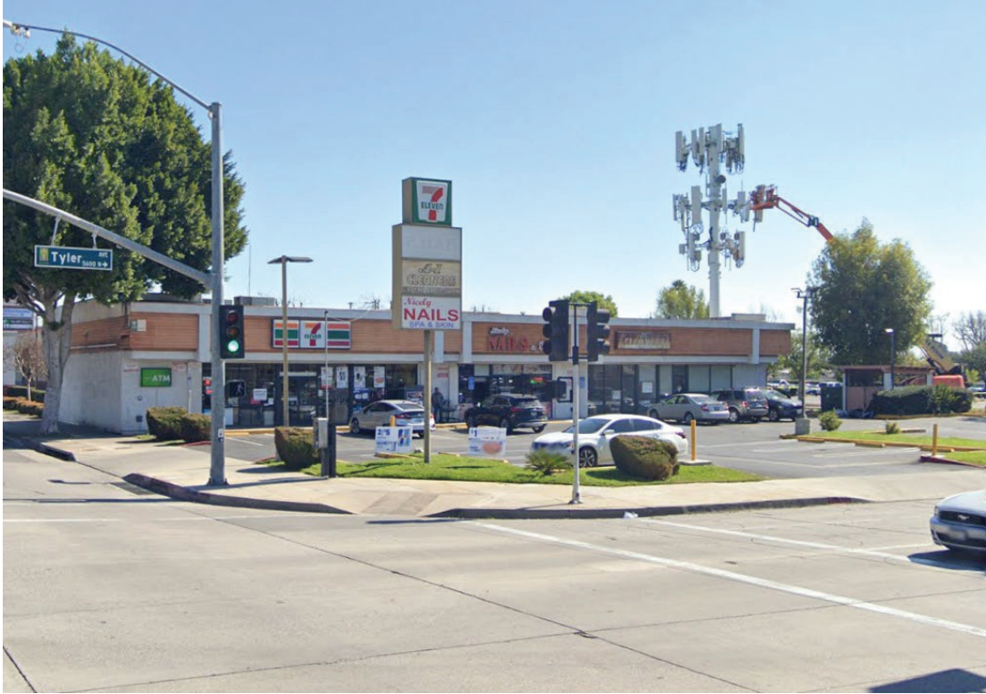
Commercial Center from the Corner of Live Oak Ave and Tyler Ave
